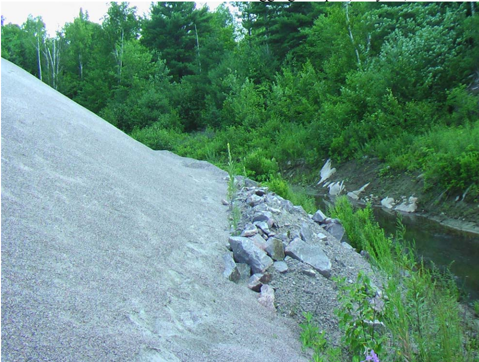
Photo 6 Stream at risk from erosion of aggregates pile, July 15, 2006
